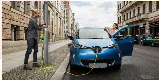
Fig.13. Charge Points From Electric Lighting Pole [16]
